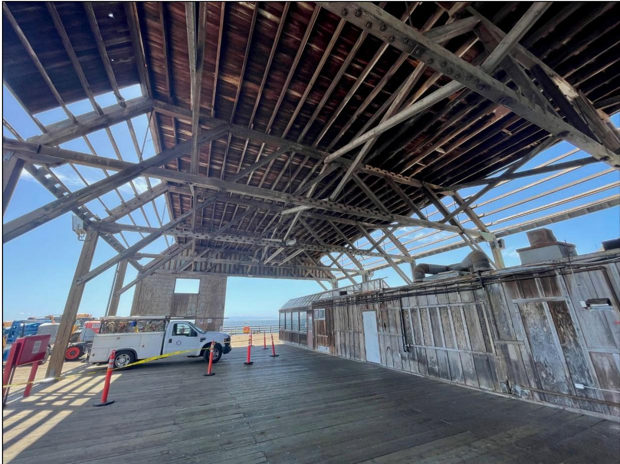
**Figure 2: Harford Pier Canopy with T&G removed to replace purlins**
